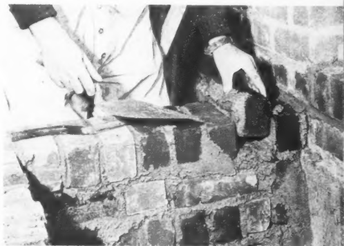
Above: Making an outside wall for steps. Bricks should be wet for best results. Below: Aligning the first step. A level, straight edge and string—plus a bit of patience—will produce a good looking and lasting job.
